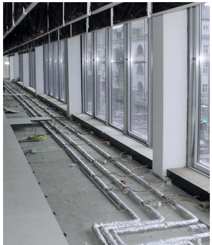
Example of double floor structure installation
